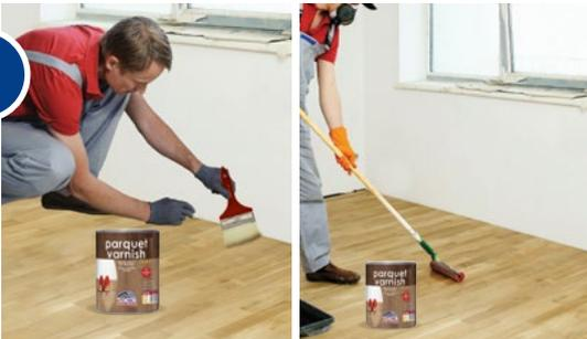
Apply the water varnish Parquet Varnish Hydro in two to three layers following the wood grain by using a brush for the “cuts” and a roller brush for the rest of the parquet surfaces.
