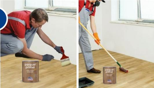
Apply Parquet Primer Hydro using a brush for the rest of the surface, one or two coats, depending on wood absorbency.
