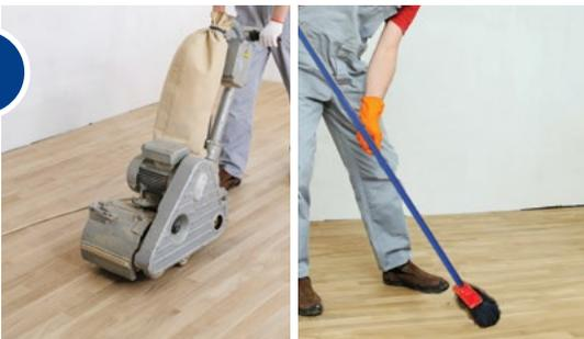
Sandpaper to completely cover wood pores and then clean the parquet well of any dust.
